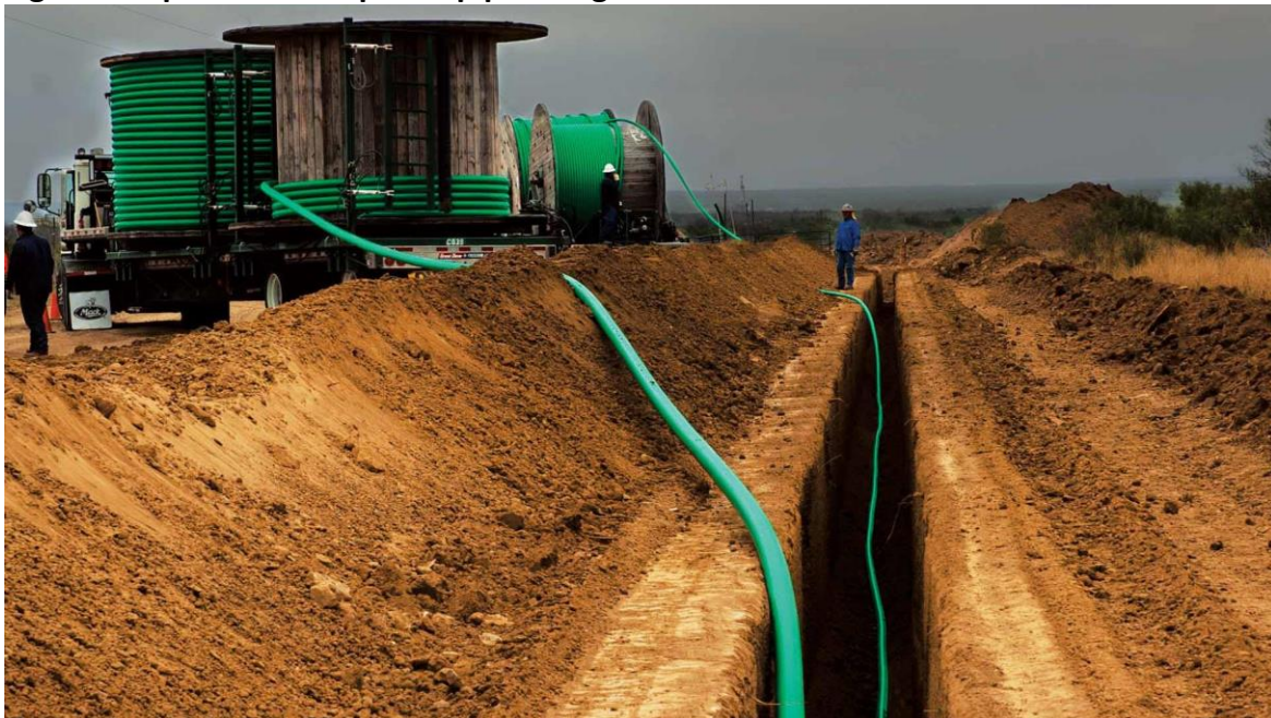
Figure 12 Spoolable composite pipe being installed
